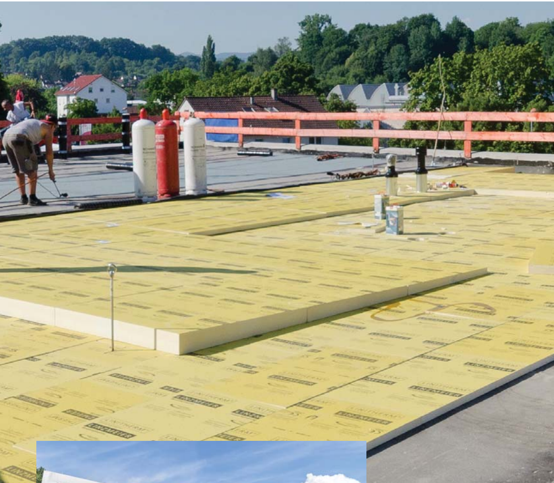
LINITHERM PGV gradient insulation Wannweil fire station
