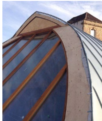
Old building restoration or new buildings LINITHERM PGV Flex common rafter insulation in combination with LINITHERM over-rafter insulation for lowest structure heights.
